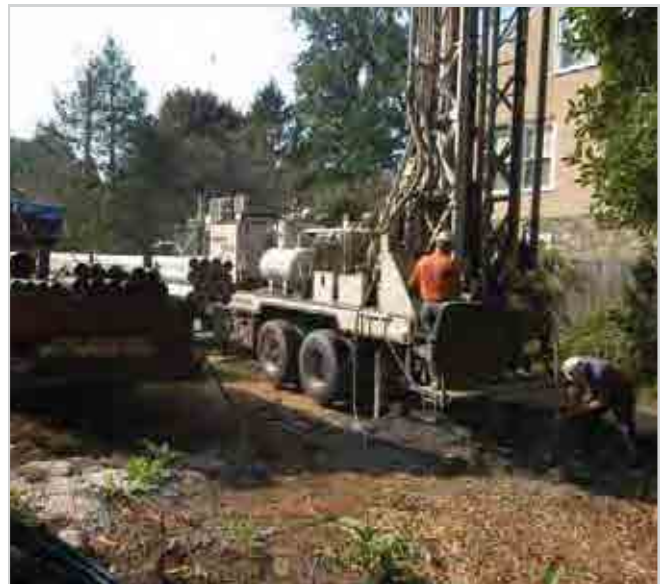
To drill wells for ground-source heat pumps, the site must be large enough to accommodate a large drilling rig.
