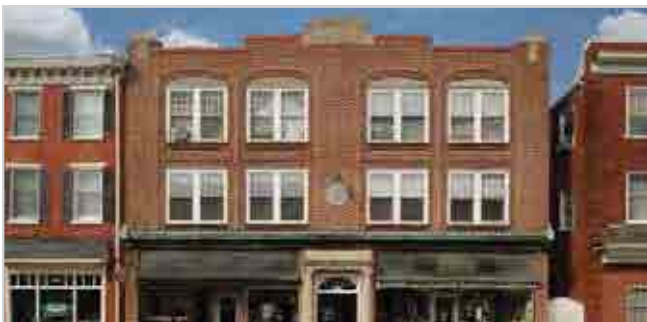
Tinted glass is not recommended for historic windows. Coatings on glass change the scale of window openings, making the wall appear more monolithic and lacking in human scale. Also, the connection between building interior and the streetscape is lost.
