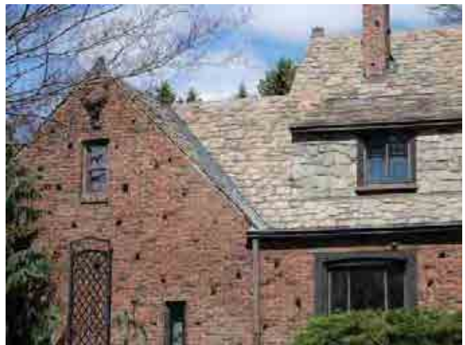
300 River Road, designed by John H. Craner in the Tudor Revival Style. The ragged-butt style slate roofing and dormer wall siding along with the clinker bricks used in the brick walls reinforce the image of the rustic cottage.
