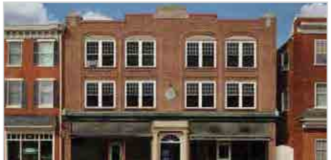
Tinted glass is not recommended for historic windows. Coatings on glass change the scale of window openings, making the wall appear more monolithic and lacking in human scale. Also, the connection between building interior and the streetscape is lost.
