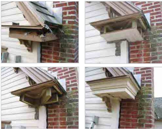
Sequence of restoration of a severely deteriorated cornice return. The crown molding was custom-cut for the project, a procedure that requires scheduling but does not add significantly to the repair cost.
