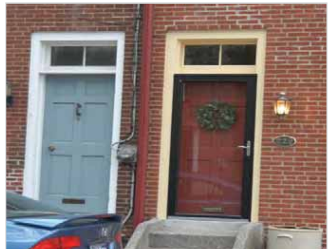
When a storm door is required to further protect the front door opening, the storm door design should be simple and should allow the historic door to be visible. While wood storm and screen doors are preferred, simple aluminum doors that are finished with a baked enamel finish are also acceptable. Scalloped edges and cross-buck patterns on aluminum storm doors are not appropriate.
