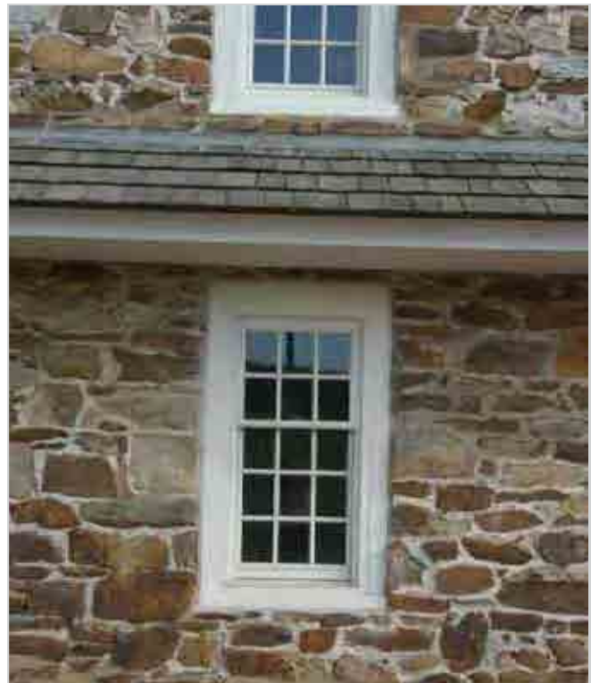
Standard size vinyl replacement windows fitted to window frames by means of wood filler strips destroy the original proportions of the windows and are not recommended.
