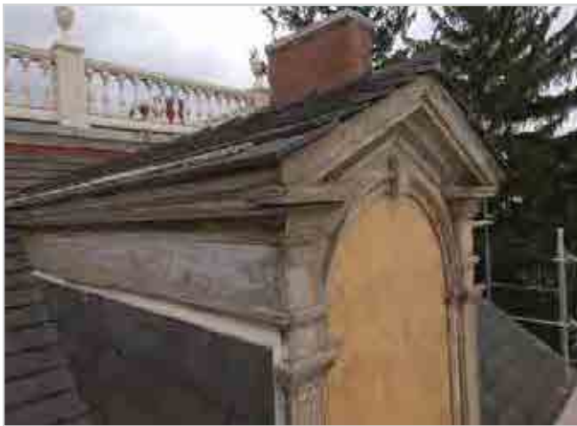
Despite inconsistent paint maintenance, the durable, old-growth heart pine used in the 200-year old moldings of this dormer are repairable, accept paint readily, and offer a more reliable service life than new woodwork. Left: Following paint removal and prior to woodwork restoration; right: completed dormer.
