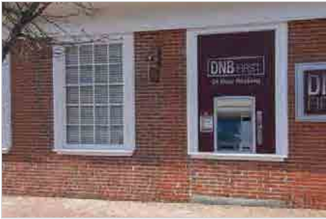
ATM machines should be installed in existing masonry openings so that the installation is reversible.
