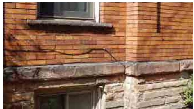
Ochre-color mortar was typically used for pointing the characteristic iron-spot brick of Beaver, while a tannish mortar in a raised-bead profile was used on the tan sandstone foundation walls.
