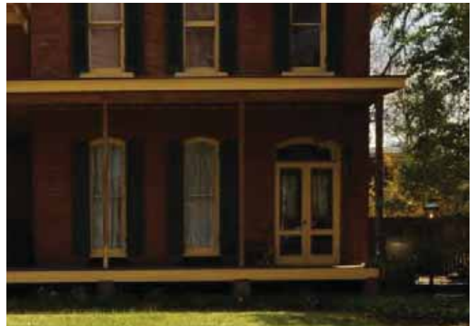
Wood storm doors that allow a view of the historic paneled wood door(s) are most compatible with a historic house. Note also a rare example of paneled shutters on the first floor louvers on the second.
