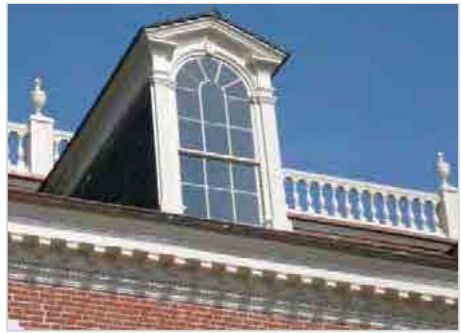
Despite inconsistent paint maintenance, the durable, old-growth heart pine used in the 200-year old moldings of this dormer are repairable, accept paint readily, and offer a more reliable service life than new woodwork. Left: Following paint removal and prior to woodwork restoration; right: completed dormer.
