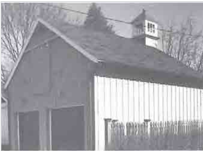
This new garage is compatible with a historic setting through its use of traditional board-and-batten siding, gable roof form, storage loft, and placement on the lot.
