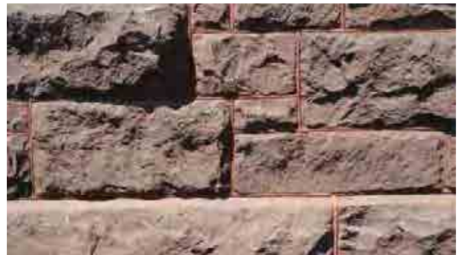
Recent raised-bead profile, tinted pointing at Park Presbyterian Church exhibits a high degree of workmanship.
