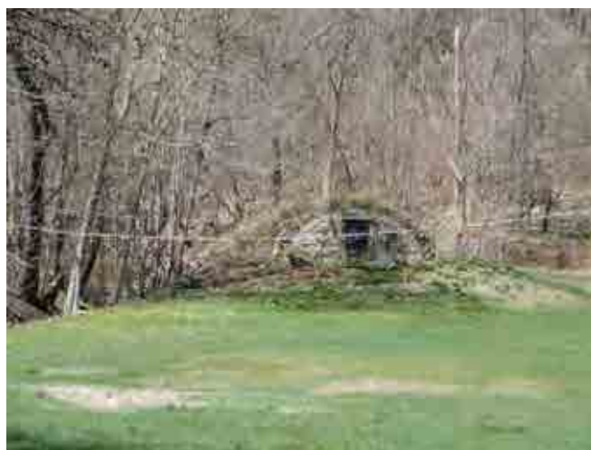
Water Lot, at the corner of 5 th Street and Wayne Street, was the source of water to Beaver Borough from 1802-1886. Springs from the hills to the north supplied water to the surviving, vaulted-stone reservoir, from where water was piped via wooden pipes to the center of town.
