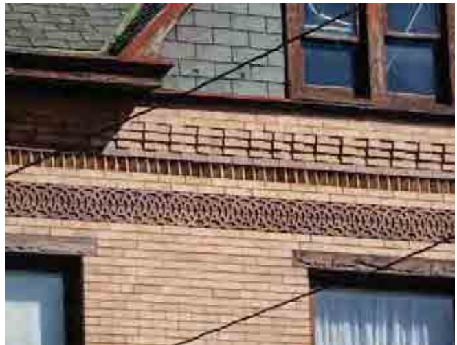
Ironspot brick is one of the most distinctive materials in the historic district. At 951 4th Street, custom brick shapes and bonding patterns are used to highly decorative effect.
