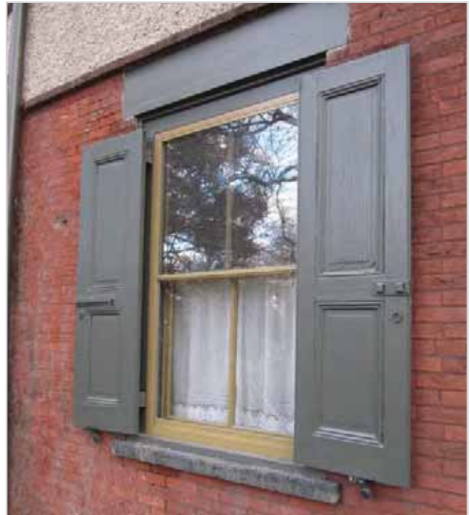
Custom-color, three-track storm windows are now available as flush units that are placed in the shutter rabbet of the historic window frame.
