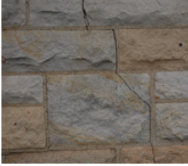
Figure 3: Cracking Mortar
