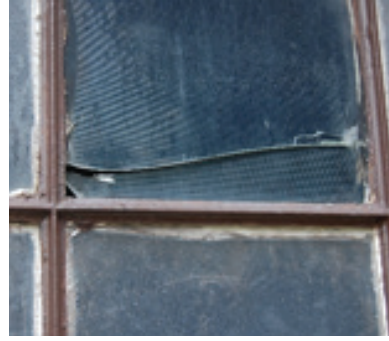
Figure 4: Cracked leaded glass
