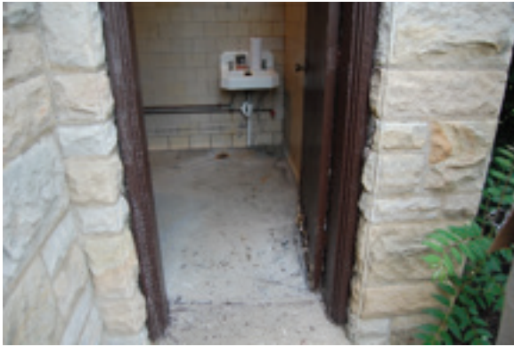
Figure 10: Width of door not ADA compliant
