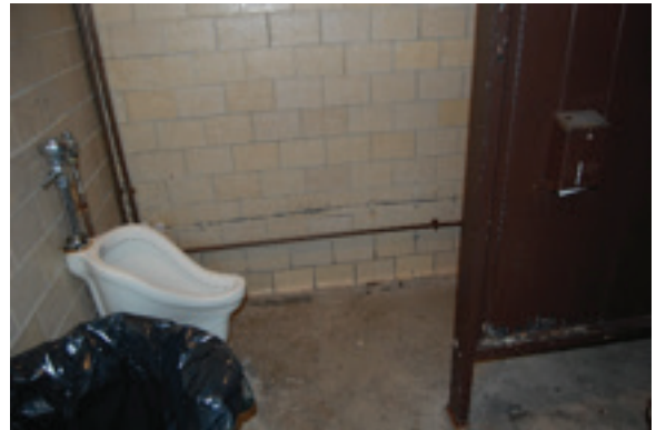
Figure 13: Urinal not ADA compliant
