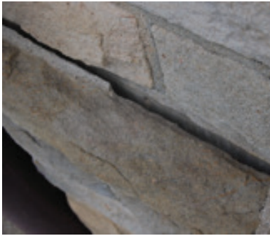
Figure 5: Separation of mortar from concrete structure
