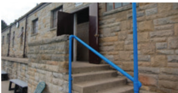
Figure 9: Large change in elevation from pool deck to bathhouse
