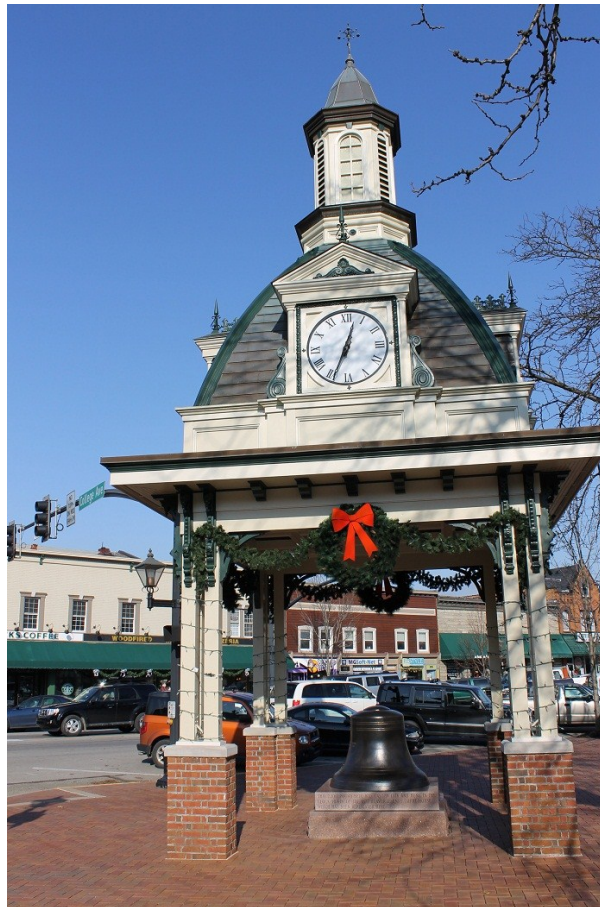
The newly cleaned and repainted 1877 Clock Tower on the corner of College Avenue and Third Street. (Photo by Valentine J. Brkich)
